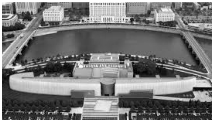
The new COSI building, including Central High School
